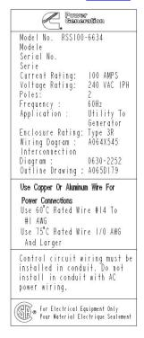
FIGURE 5. RSS100 WITH CONTROL DISPLAY NAMEPLATE
