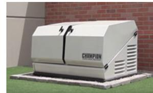
A concrete pad can be poured and the HSB secured to it. In some areas a concrete pad is required due to high wind potential. Check local codes to see what type of mounting base is required. If a concrete pad is required, all federal, state and local codes should be followed. Unless mandated by federal, state or local code, a concrete pad is not required.
